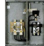
EXAMPLE 400 AMP METER SOCKET LOAD CENTER
