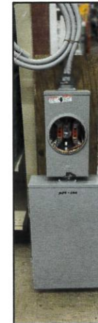
PRE-ASSEMBLED EXAMPLE METER SOCKET WITH DISCONNECT
